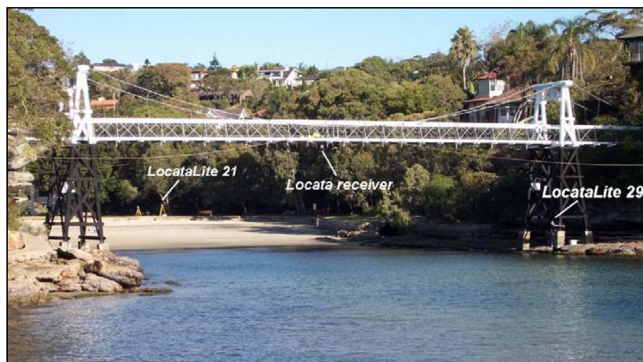
Figure 4: Parsley Bay suspension footbridge trial using Locata .
