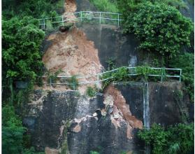
the subject slope was potentially hazardous but more detailed information on the slope movement was required to determine whether to exercise emergency evacuation. SD was called upon to monitor the slope and provide timely results to the engineering counterparts.
