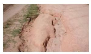
Figure 3: The erosion phenomena on the main settlement access road.
