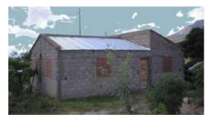
Figure 8: Informal house, with cement block walls and roofed with iron sheets.
