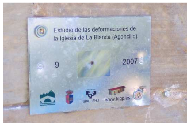
Figure 4 - Plate with information about the project and nail (bottom right).
