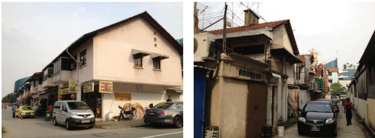
Figure 5: Features extended from building walls.
