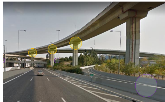
Figure 2. Test bridge. The inclinometer locations on the piers and ground are circled in yellow and purple.
