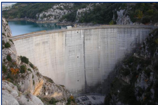
Figure 1. Sainte Croix arch dam
