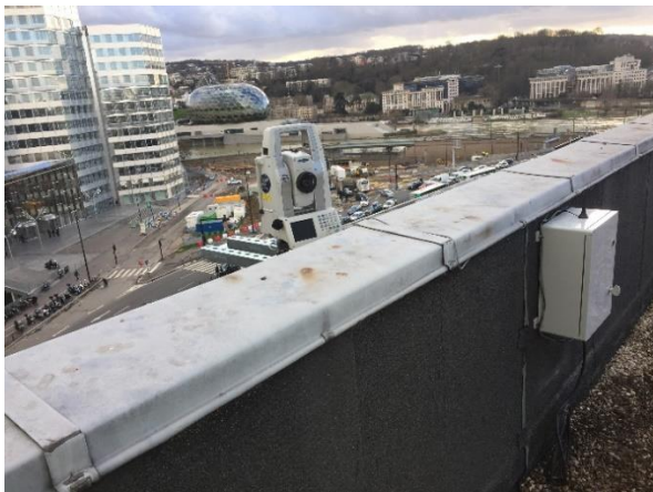
Figure 2. Robotic Total Station for monitoring buildings on line 15
