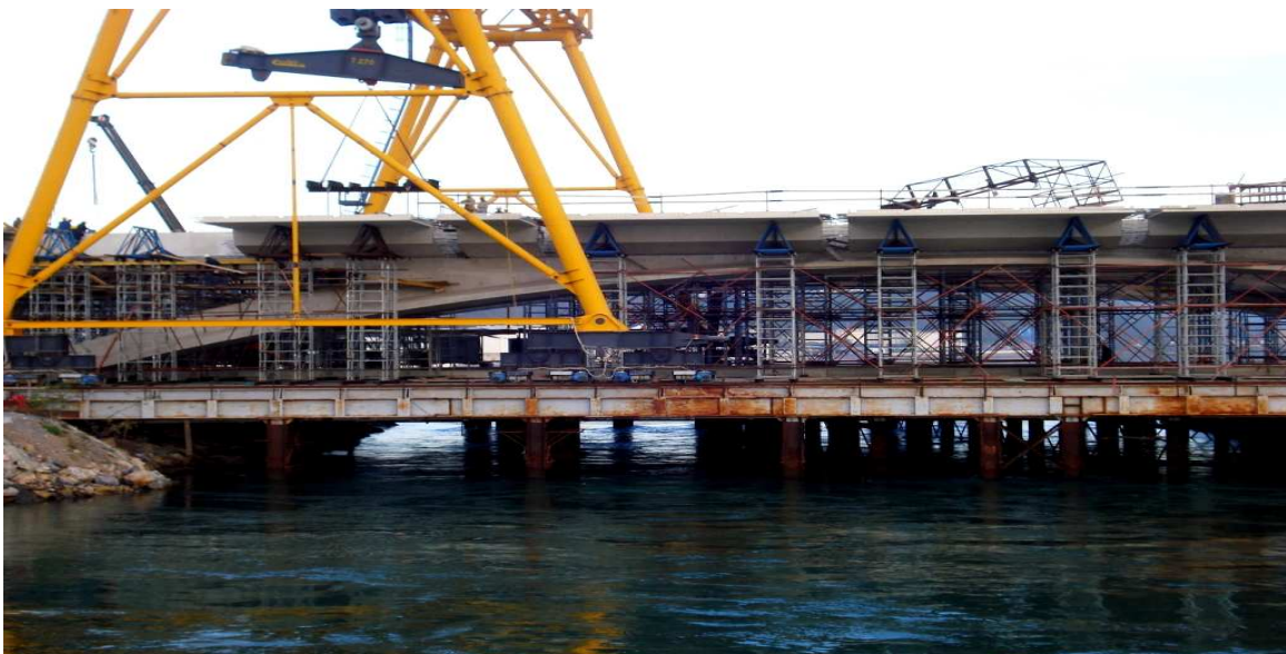
Figure 18: Pose des demi-caissons.
