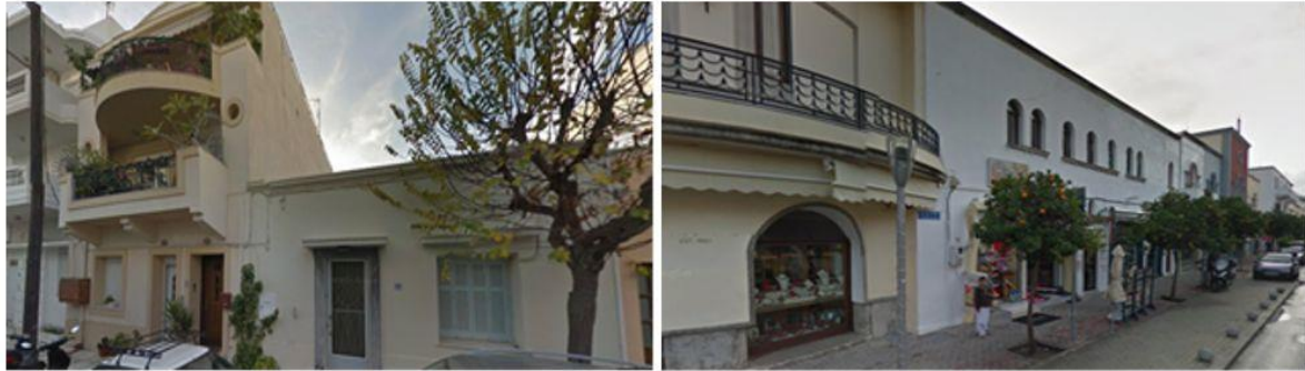
Figure 3 - Typical examples of residential buildings in the area
