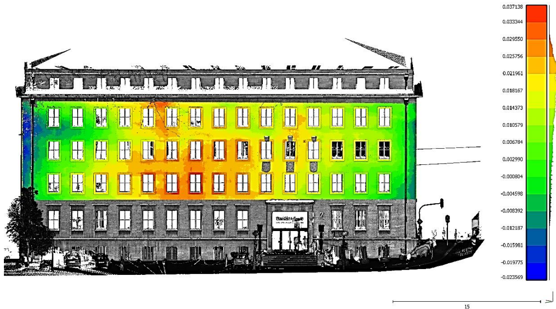
Fig. 4. The deviations field for comparison CAD and point cloud model The first comparison we made in the most traditional way. It is comparison between CAD model and point cloud. The results of this comparison is presented on fig. 3 in the form of deviations field.
