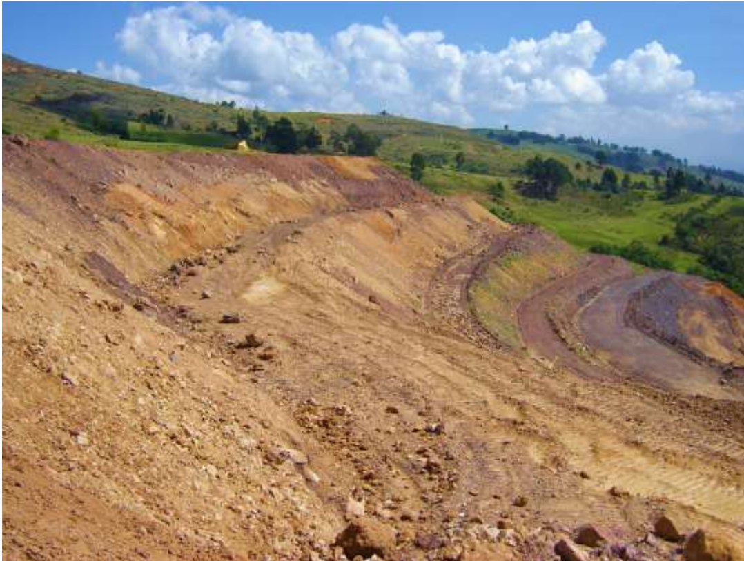
Geometric conformation of sterile disposal area and subsequent geomorphological restoration.
