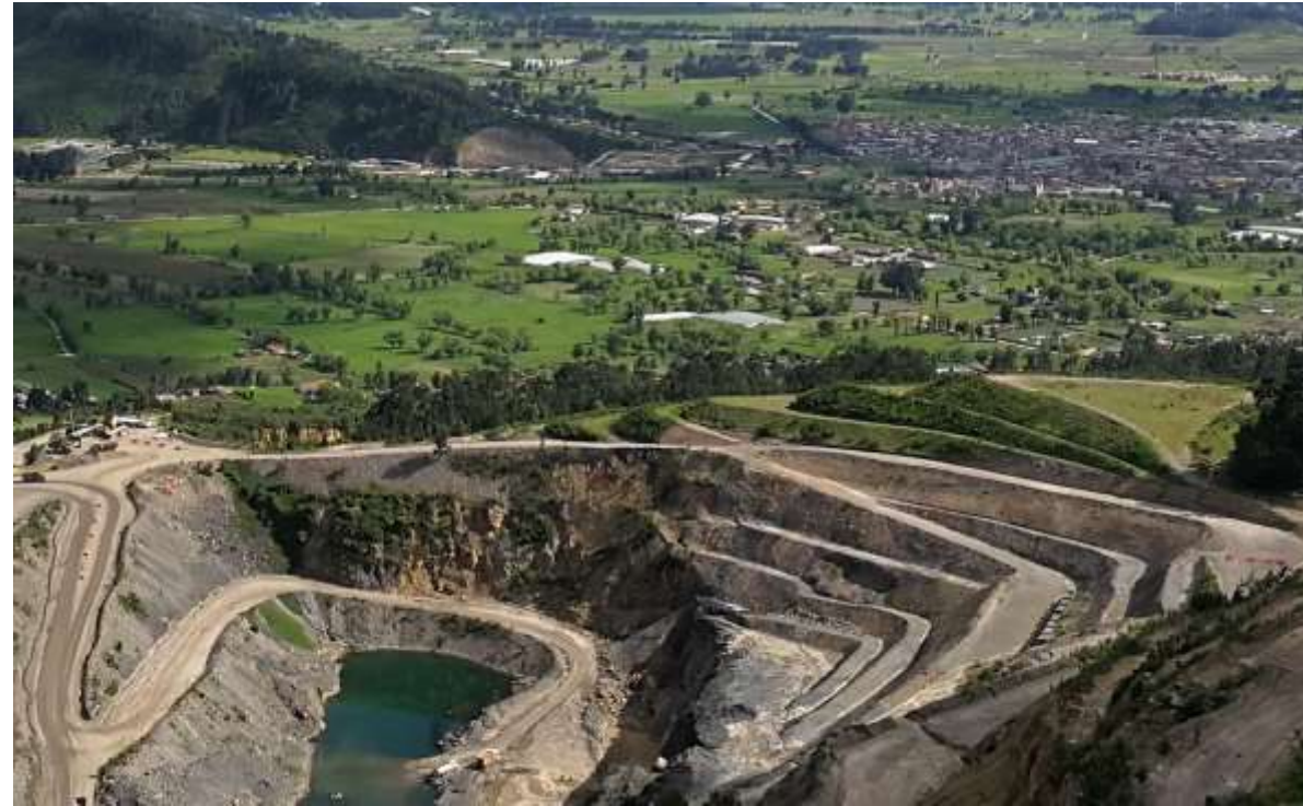
Design of terraces of constant height and berms in a single nibe
