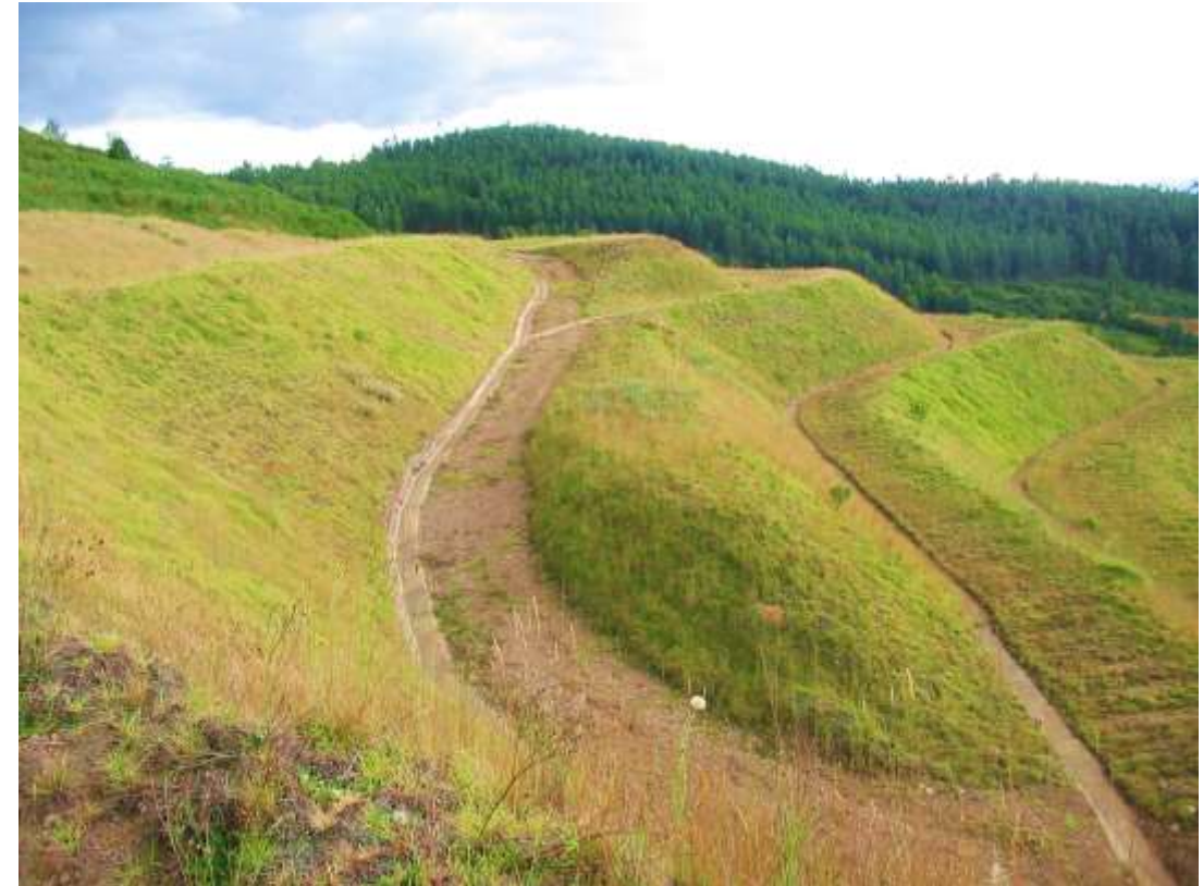
Geometric conformation of sterile disposal area and subsequent geomorphological restoration.
