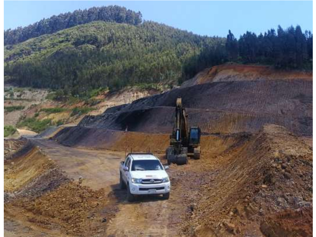
Geometric cut with heights and widths of berms established in the design.
