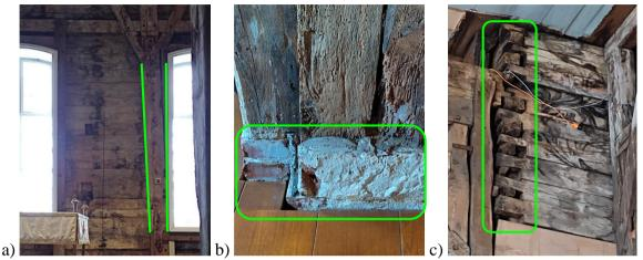
Fig. 2. Visible weaknesses in the structure of the church: a) the columns of the original frame structure significantly inclined towards the entrance (west), b) the brick base of the column, which was originally entirely wooden, c) weakened connections of the carcass structure
