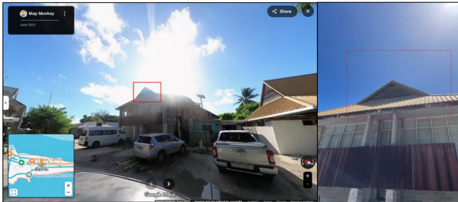
Figure 4: A-frame fascia of the Bairiki LMD building (street view and close-up)
