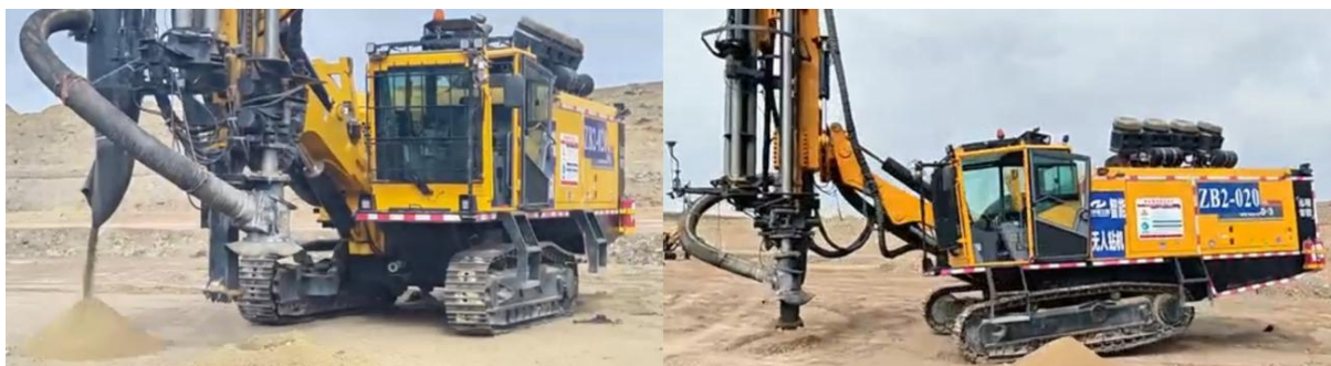
Figure 11-Application at Job Site
