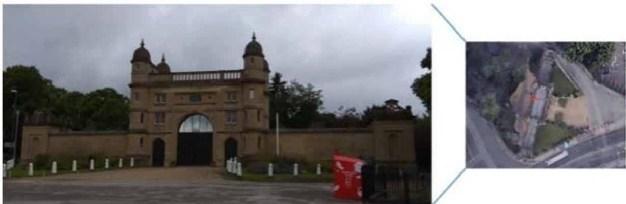
Figure 6 Old building located on the derby Road, Nottingham.
