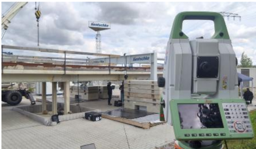
Control measurements using a total station (Bautzen)
