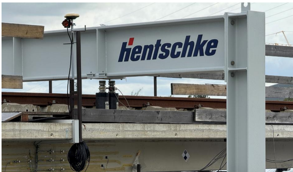
GNSS antenna with integrated prism (center); total station used for control measurements (right)
