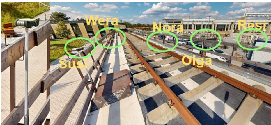
Abb. 2: Mounting of the five antennas in the research project, along with their assigned names
