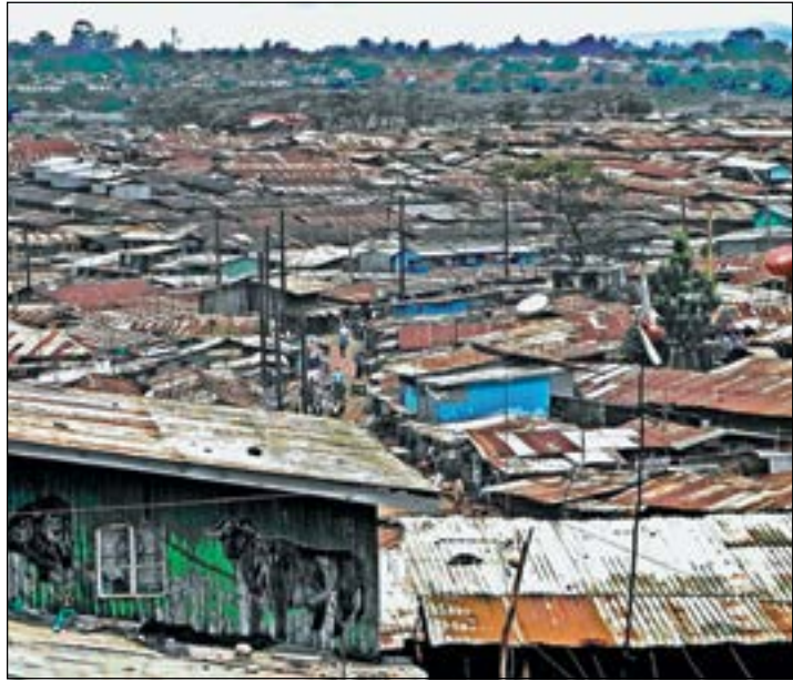
Figure 7.4 The informal settlement of Kibera in Nairobi, Kenya, houses 1 million-plus people in an area of 150 ha, or about 0.6 sq. mi.
